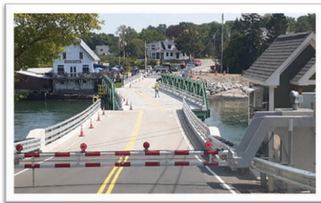
The Grand Opening Ceremony for the new Barter Island Bridge was held on August 2, 2021. Joan Hodgdon and Evelyn Shahan cut the ribbon and a skit was done replicating when the neighborhood children would all run to open the old bridge. Roland McLellan was the first to drive over the new bridge with Stanley Hodgdon as copilot.
